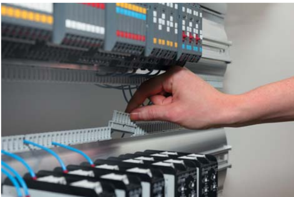
Step 1: Release the comb unit
