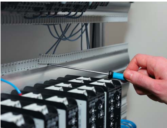
Step 1: Release the combs with a screwdriver
