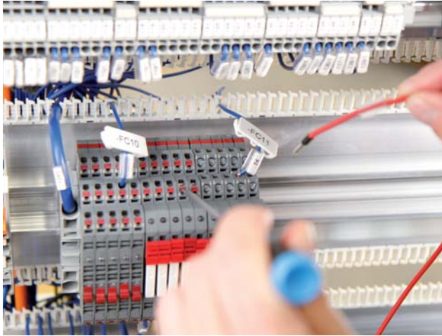
Step 1: Connecting the wires to the components
